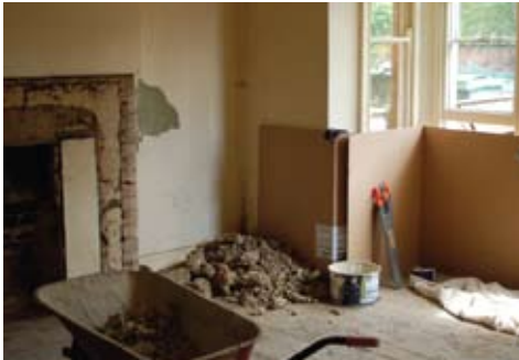
■ Refurbishment work in progress
